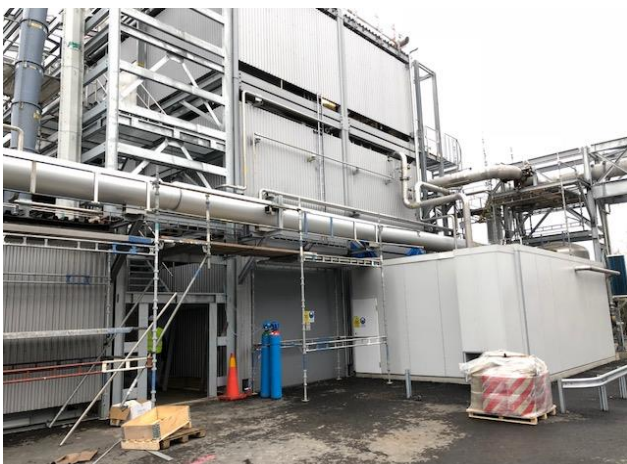
The compressor room is seen to the right in the picture
