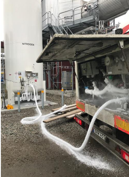
Filling of the nitrogen tank
