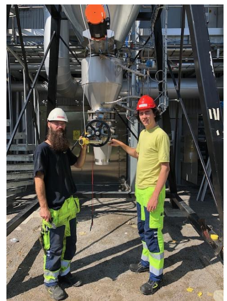
Magnus Andersson and Matthias Scrive deploys a level guard to control the level of ash in the filter.
