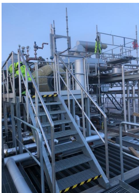
Welding work on top of the gasifier
