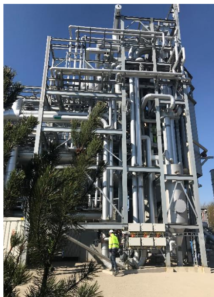
Steam system, which been covered with scaffolding until April
