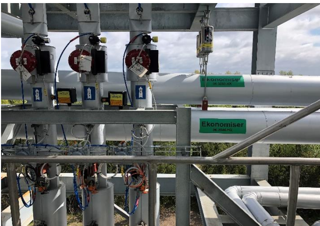
Labeling of pipes is an important detail in the "finishing work".
